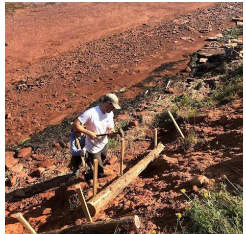
Living shoreline installation (2021)
