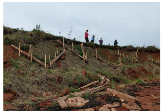
Living shoreline installation (2021)
