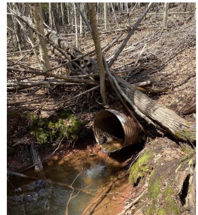
Example of a hanging culvert in Stratford.
