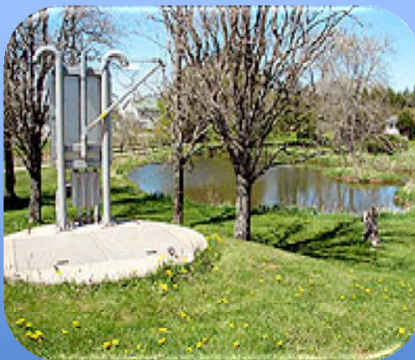
Figure 8: Sedimentation ponds are used in drainage systems as means to alleviate flash floods, in Stratford, PEI.
